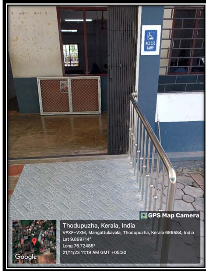
Ramp 4 with Rail
